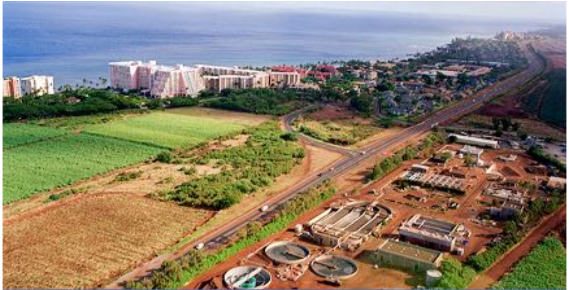
Maui County, Hawaii, wastewater treatment facilities at issue in Supreme Court litigation. Credit: Warren Gretz/NREL via E&E News.
